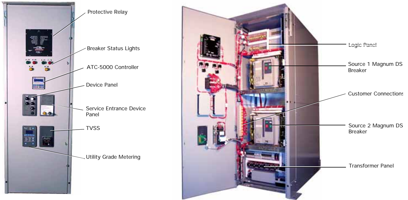
Figure 5. Magnum Soft Load ATS Base Components.
