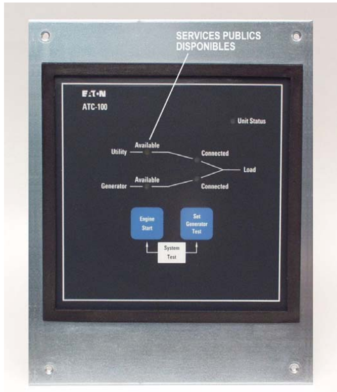
Figure 18 – Logique ATC-100 (Services publics alimentant la charge)
