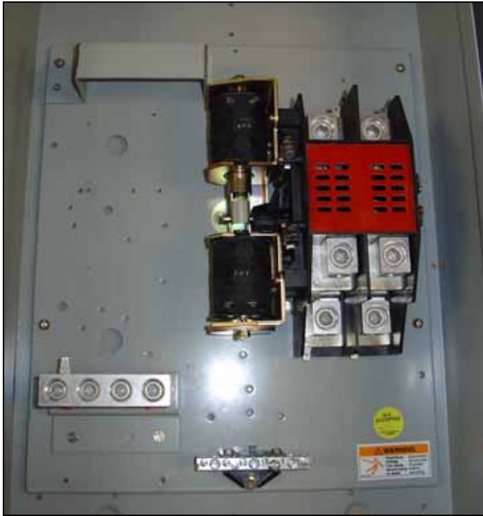
Figure 4. An RLC1 200 A Standard ATS.
