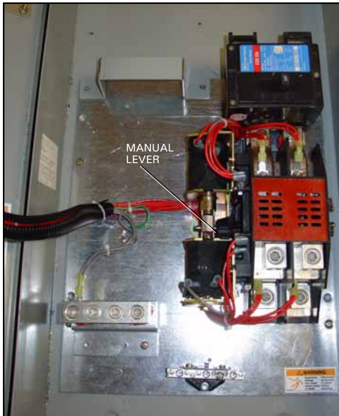
Figure 23. ATS Manual Operating Handle in Use.
