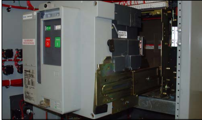
Figure 14. Drawout Mechanism (Closed Transition Shown)
