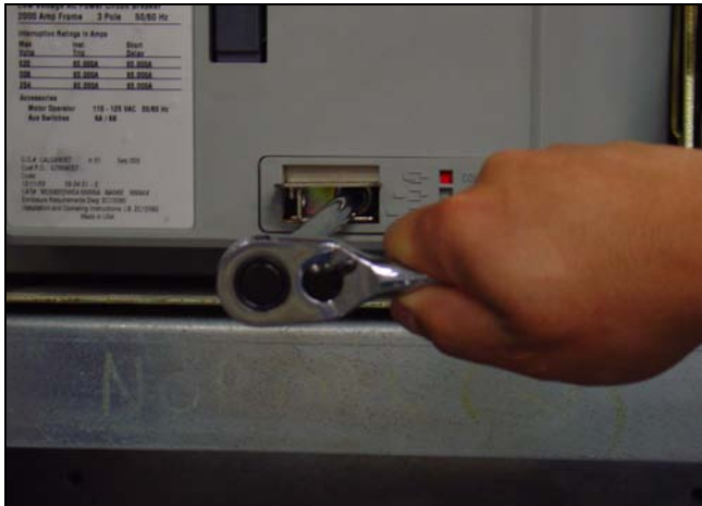
Figure 33. Levering and Position Indication.
