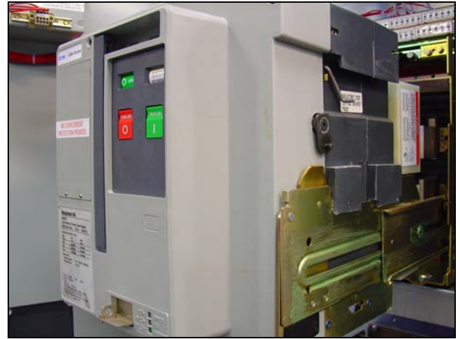
Figure 9. Drawout Switching Device Fully Extended from the Magnum Transfer Switch.
