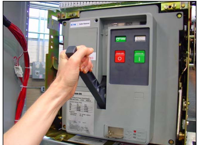
Figure 23. Pumping Handle Charges Stored Energy Mechanism (Closed Transition Shown).
