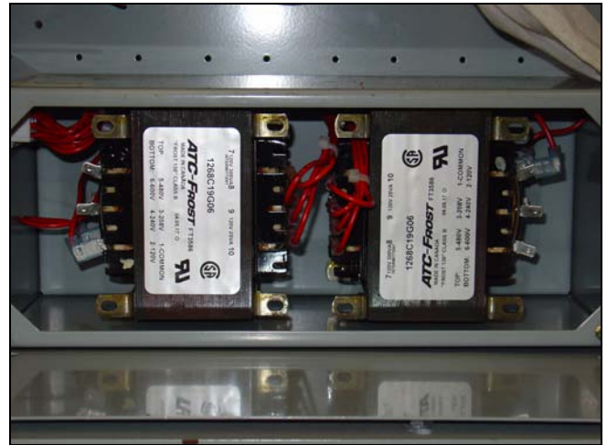
Figure 16. North American Market Voltage Selection Terminals (Shown Connected to the 120 Vac Taps).
