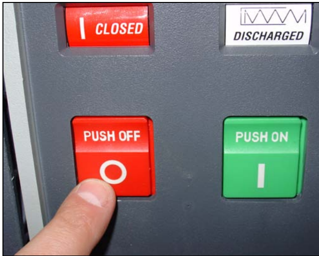
Figure 24. Close Switch by Pushing Close Button.
