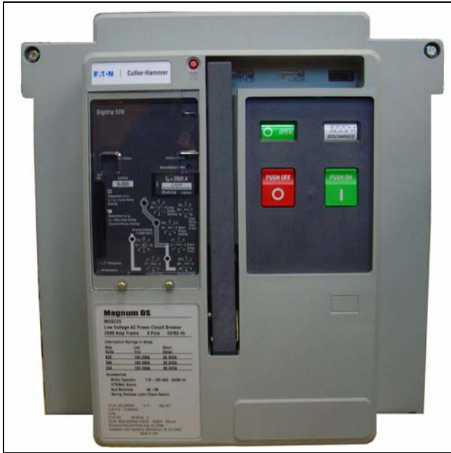
Figure 7. Fixed Switching Device for the Magnum Transfer Switch.
