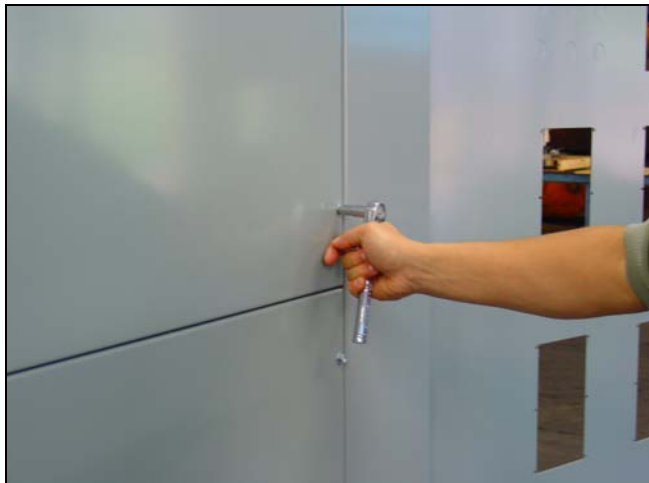
Figure 39. Removing the Bolts
