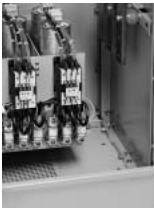
Bottom Entry Location
